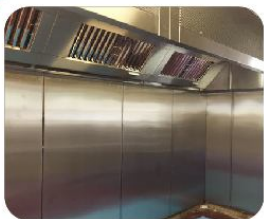
SS Wall Cladding
