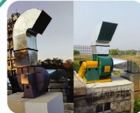
Belt Drive Centrifugal Blower
